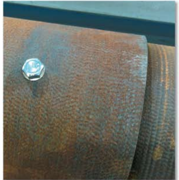
Poles have press-fit joints which are loaded in a hydraulic press and pinned with a mechanical fitting.
