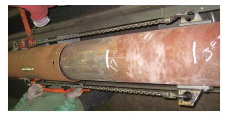
Pictured Above: Four jacking lugs are attached with bolts provided with the McWane jacking kit. Chain hoists are connected to jacking lugs and in position for section assembly. The 17" mark indicates the minimum section insertion amount for the example pole, which along with the B axis will be clearly marked by the factory. The minimum insertion amount will be based upon pole length and section number. The inserting section should be inserted to the minimum overlap mark.
